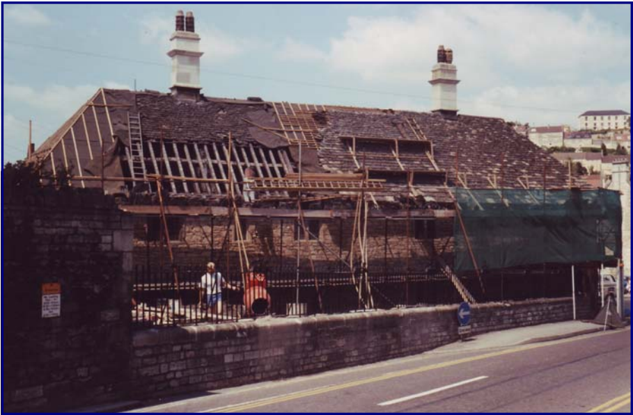
Re-roofing the almshouses, ca. 1989.
